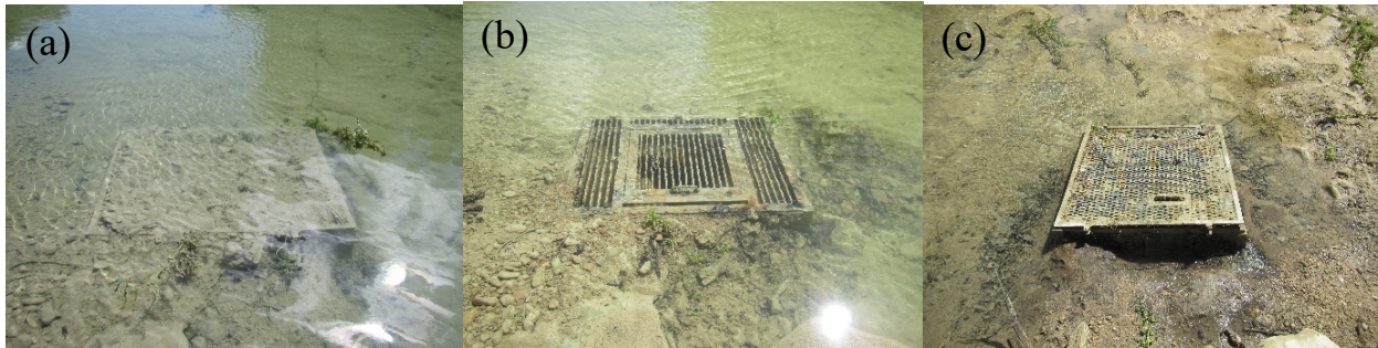
Figure A1.2: Sequence showing (a) cave gate sealed with organic debris after flooding, (b) mesh covering removed for cleaning, and (c) mesh covering reinstalled after cleaning.
