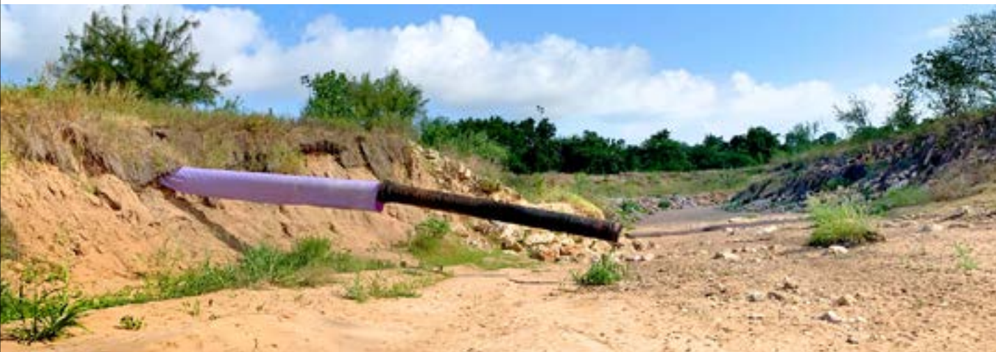
Broken reclaimed water pipe at Roy G. Guerrero Colorado River Metropolitan Park. Repairing and protecting damaged Austin Water infrastructure has been one of five temporary projects completed before the Capital Improvement Project was finalized.
