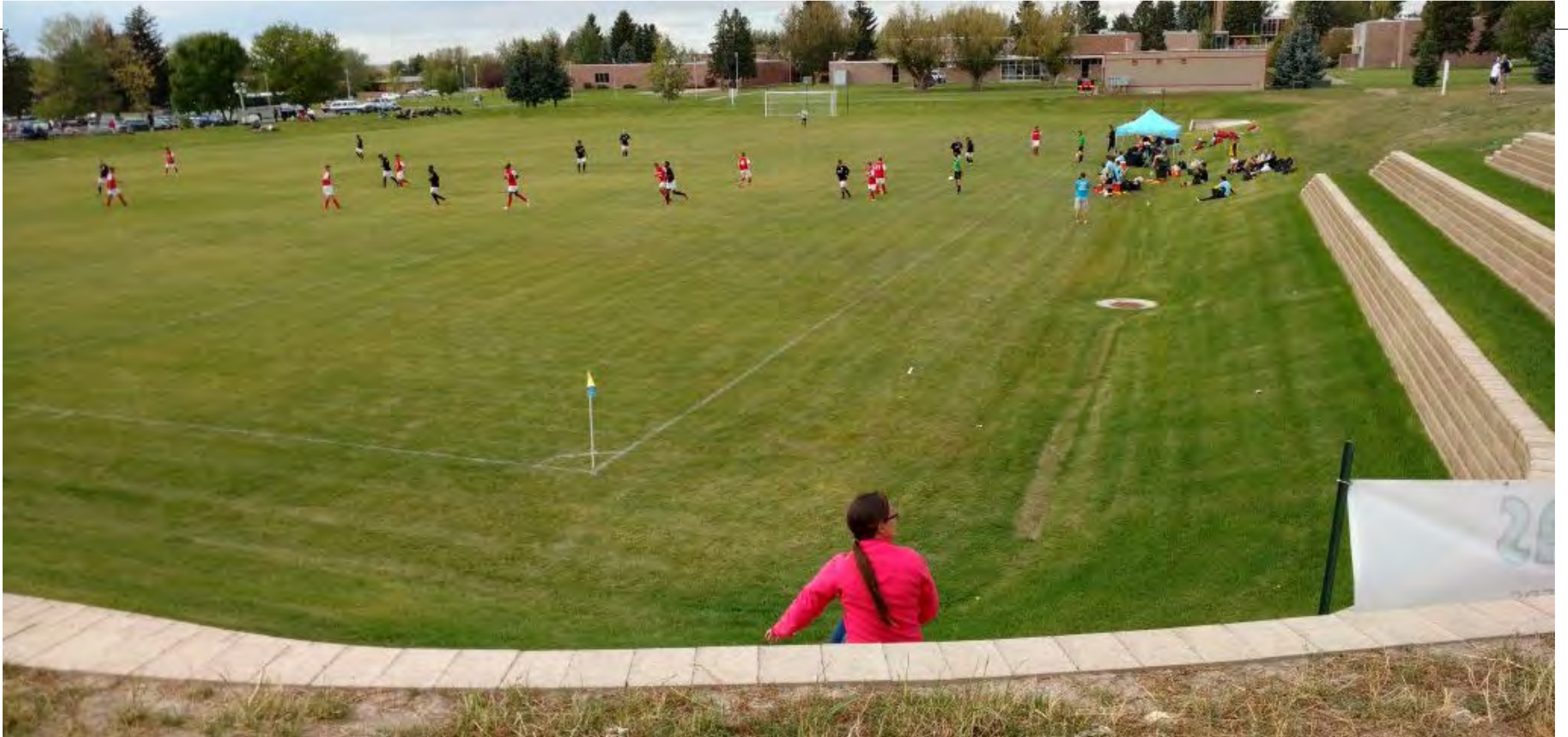
Photo credit: The Multi-use Athletic Field and Intermittent Storm Water Detention Pond by TD&H engineering in City of Great Falls, Montana
