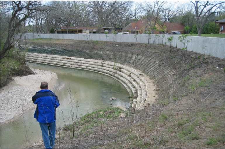
Floodwall during normal (above) and flood (below) conditions
