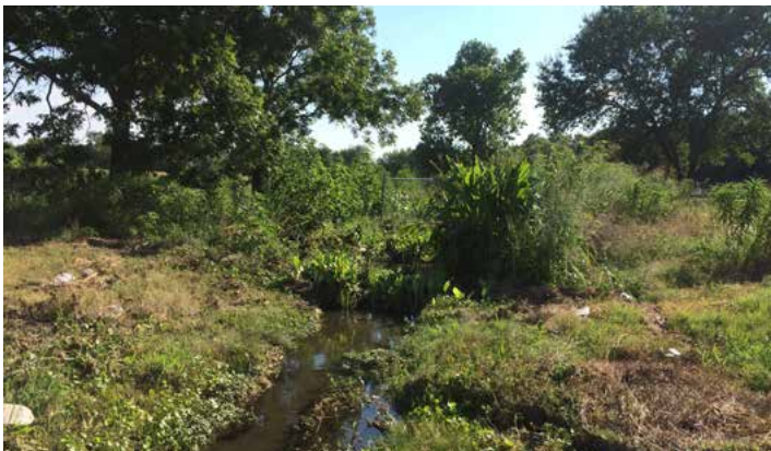
Oak springs trickle channel: mowed area before restoration in 2014 (top), channel reconfiguration (center), and two years after construction in April 2016 (bottom). Straight concrete channel in mowed area removed and reconfigured into a meandering channel with native plants.
