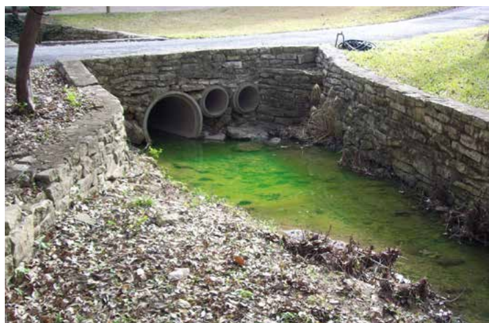
Water quality testing of this culvert in the Taylor Slough South watershed indicated high bacteria. Fluorescent green dye and smoke testing by Austin Water helped identify the source of the failing wastewater line to ultimately resolve the problem.
