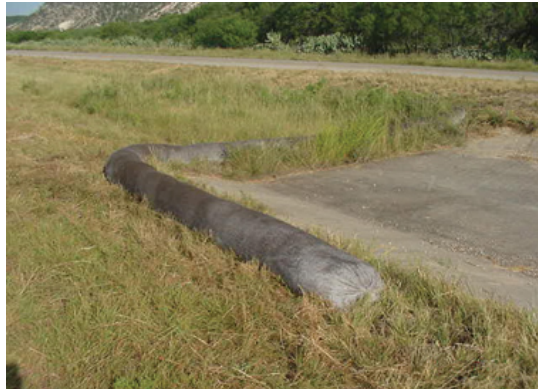
Mulch socks have proven to be an effective way to capture sediment where silt fencing is impractical. This is a photo taken on I10 near Junction, TX.
