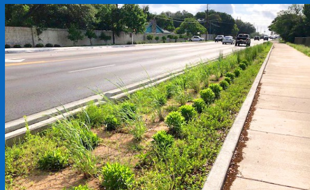
Watershed Protection installed rain gardens as part of the Anderson Mill Road Regional Mobility Improvements to improve water quality in Lake and Bull Creeks. Part of the 2016 Mobility Bond Program, this project was designed to reduce congestion and enhance safety for all road users, including people riding bikes, walking, driving cars, and accessing transit in the area.
