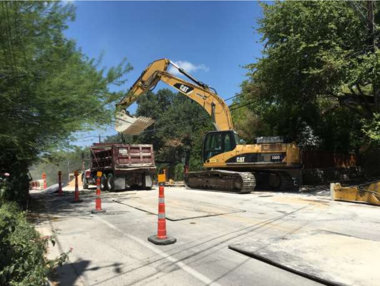
Trenching and Installation of Storm Drain Pipe
