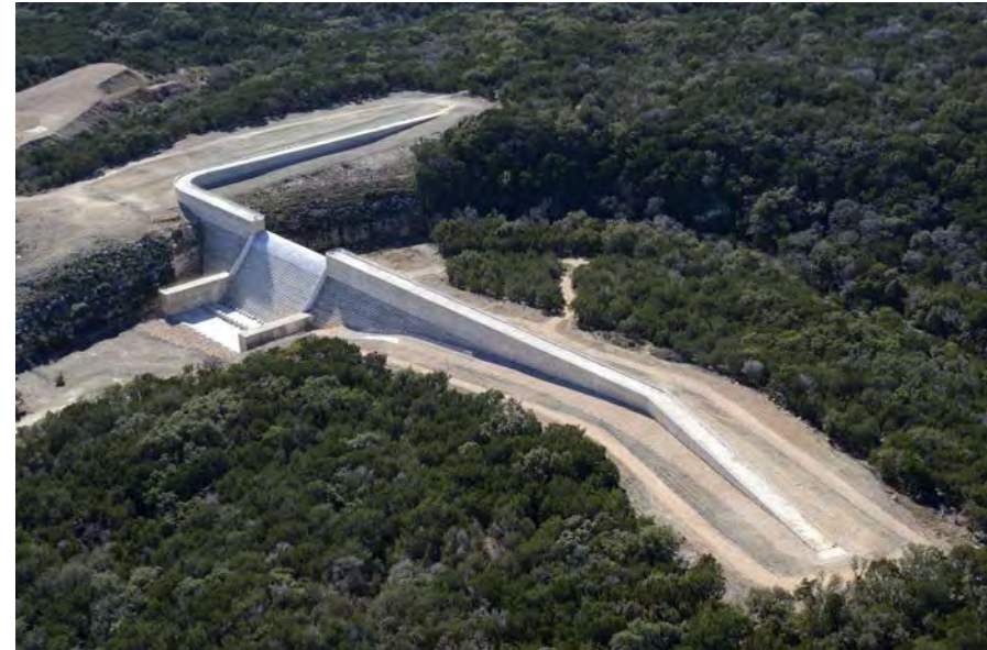
Dry Comal Creek Dam, Comal County / ~$20M / ~2,900 ac-ft
