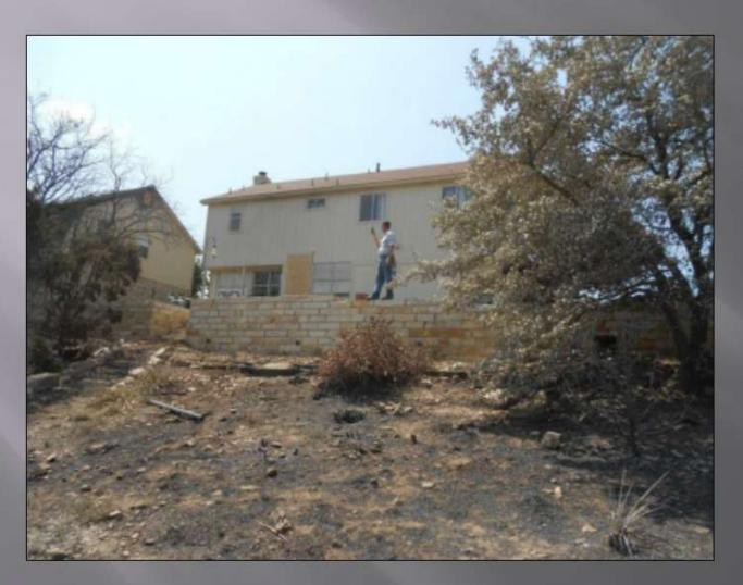
Retaining Walls can act as a vertical barrier that interrupts the continuity of fuels
