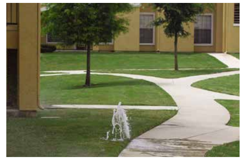
Broken spray head
