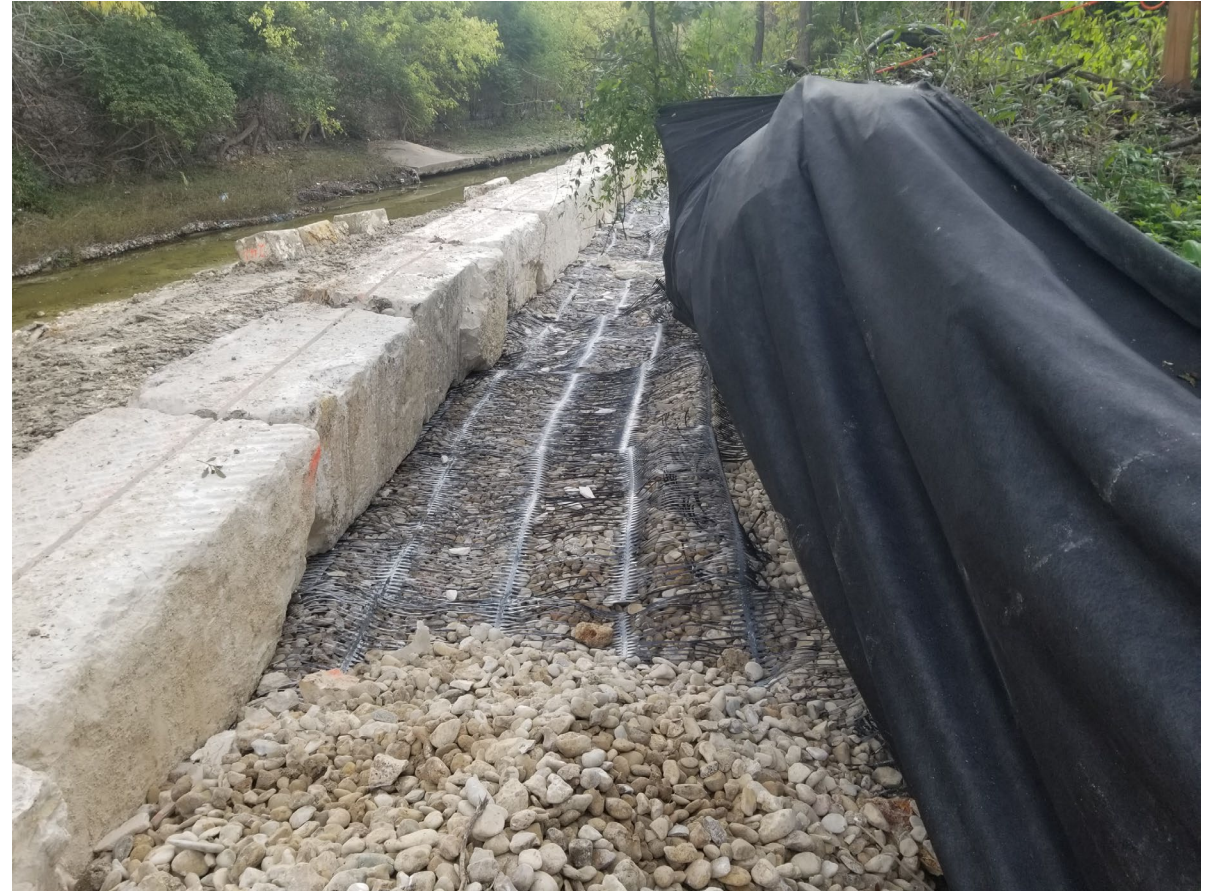
Example of MSE Block Wall
