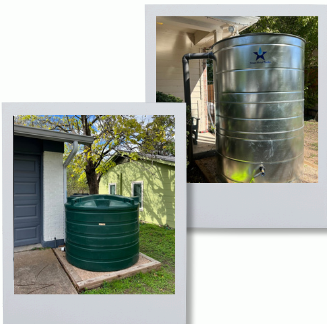
Figure 3. Examples of cisterns used in RCPP projects
