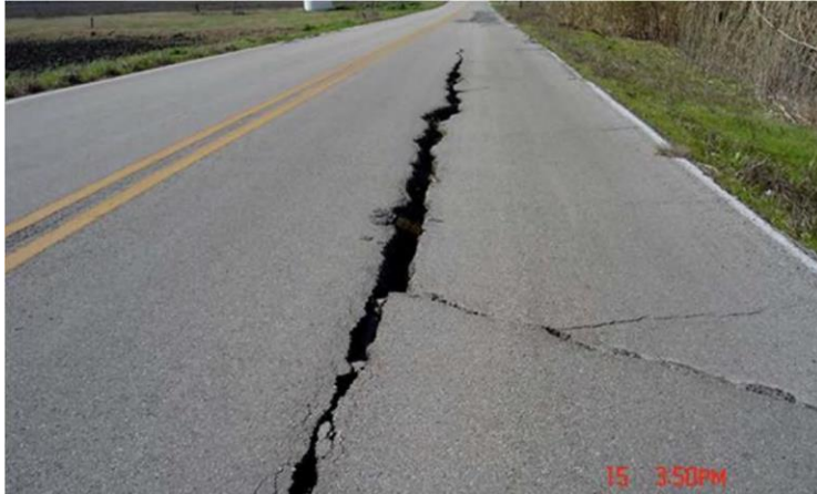
Photo of a severe pavement crack on Hamann Lane in Travis County in 2005. Photo credit: City of Austin.
