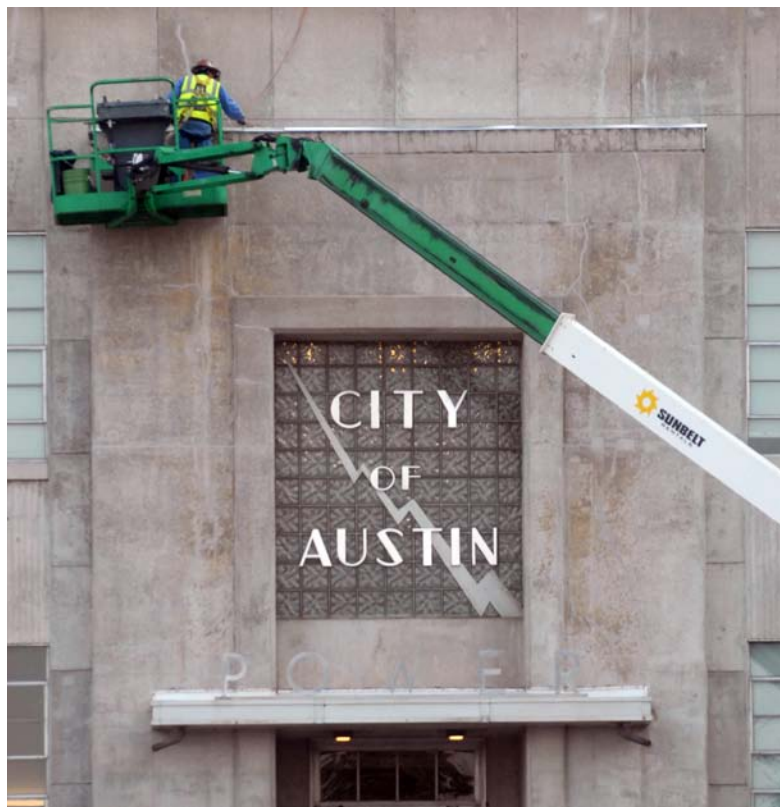
Reconstruction work on the Seaholm Power Plant.
