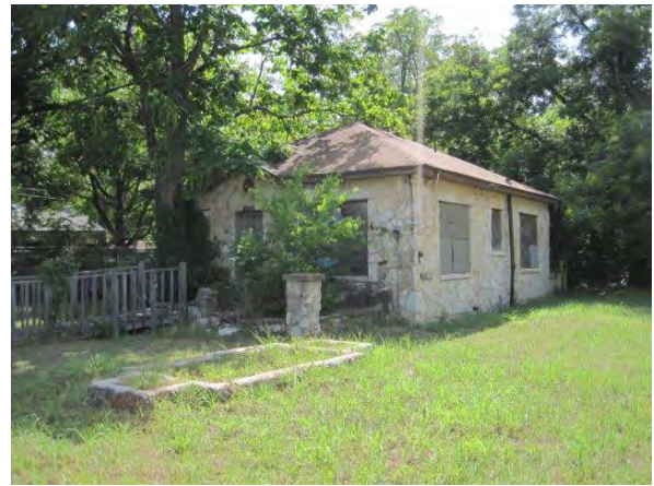
Typical view of non-contributory improvements, facing northeast from Tillery Street
