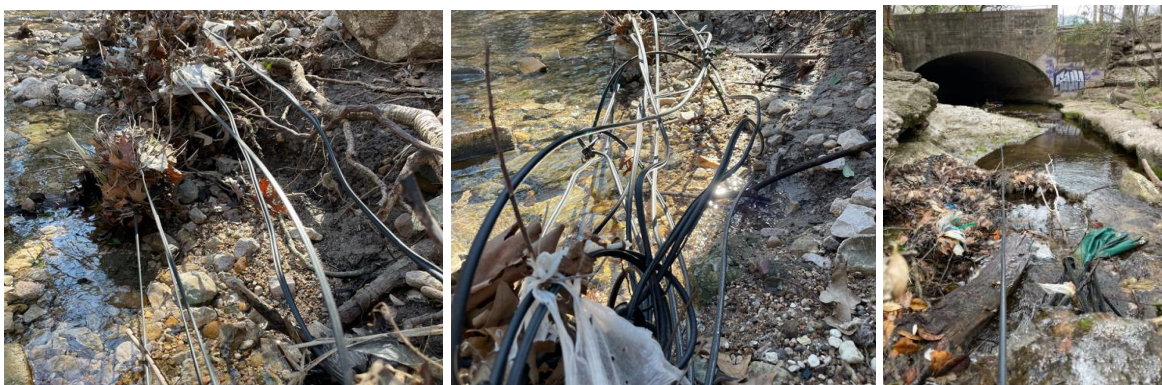
Figure 27. Telecommunication cables were a common, preventable, and significant issue in some stream reaches. Thousands of feet of internet cables were observed in discarded in creeks, some still partially attached, likely disconnected on one end by service contractor during a change in service.
